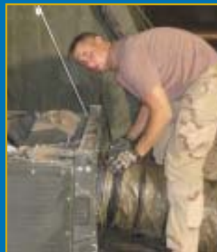
TSgt Andrew Lape, a security forces technician connects a field deployable environmental control unit (air conditioner/heater) to an Alaskan shelter at a forward deployed location in Iraq. Courtesy photo.
